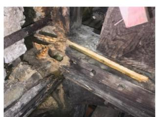
beams can be seen with the light-coloured piece of wood resting on it. The left end is the rotten part where it enters the wall. All of the rotten wood was then carved away and carbon fibre rods inserted into the end of the beam as can be seen in the lower left picture. Shuttering was then fitted to the sides and base of the beam and architectural resin poured in. After 24 hours to harden, the beam was back to full strength.
