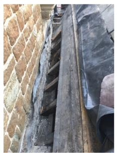
was rotten, the main cross beam was rotten where it was let into the wall and two of the three wooden supports for the beam also had rot. Time for a re-think!
